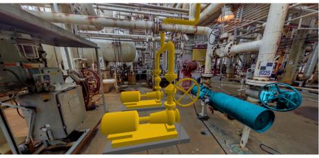
3D scan of a process plant along with imported CAD objects (image is scanned data - not a photograph)
